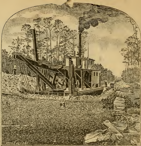
DREDGING SANTA FE LAKE, UNDER THE SUPERINTENDENCE OF NED E. FARREL.
